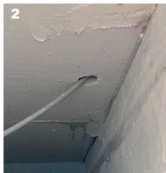
Too much space around the wiring, must be grouted.
