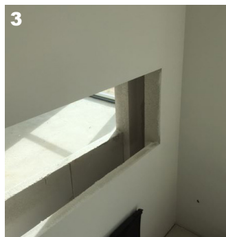
The fireplace wall is not secured against false draft in the sides.
