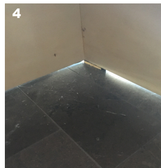
The wall is not hermetically sealed at the bottom, which can cause drafts.
